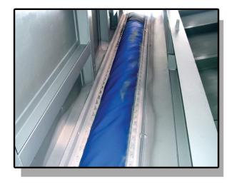
Fluoroelastomers, which are vulnerable to unpredictable chemical environments and excursion temperatures above 400°F (204°C), can be unreliable. High plant expenditures to cover the many costs associated with unscheduled or frequent expansion joint failures can be the result. Because CrossFilm™ material consists solely of PTFE resins, it is considered chemically inert in expansion joint service and is capable of performing in temperatures ranging from -400°F to 600°F (-240°C to 316°C).
