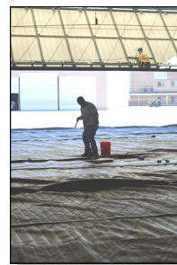
Fabrication of a large scale TCI CrossFilm™ secondary containment liner.
